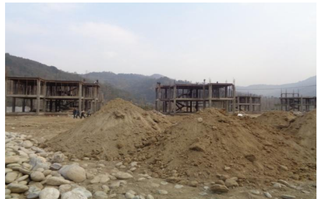
Construction of camp facilities
