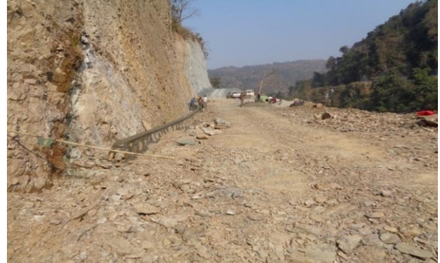
Side drain and road widening work near the powerhouse area
