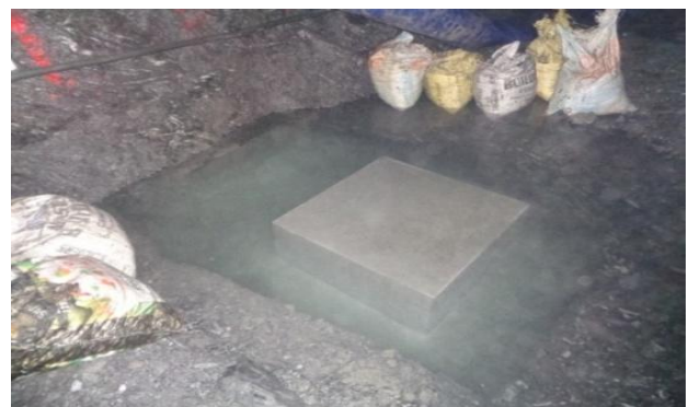
Block Shear Test preparation in underground powerhouse
