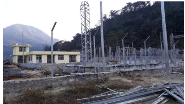
Construction power sub-station
