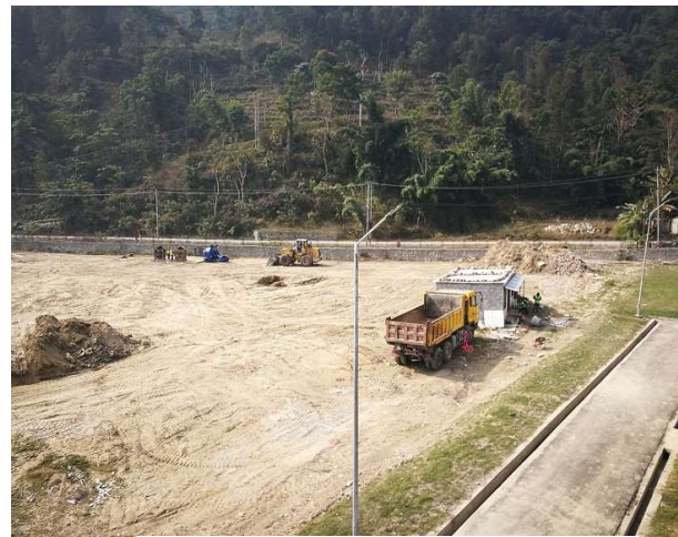
Preparation of Site Establishment Areas
