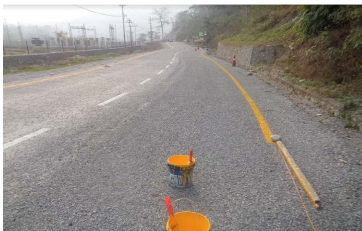
Access Road towards Power House
