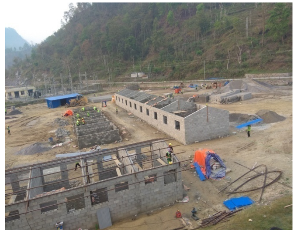
Construction of Camp Facilities
