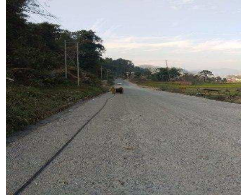
Access road towards Camp Site
