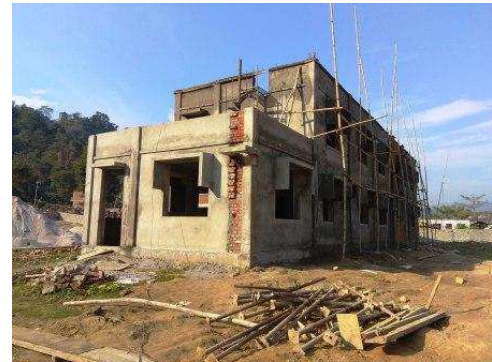
Construction Camp facility
