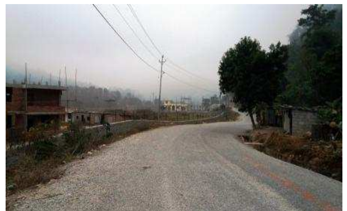
Access road towards Power House
