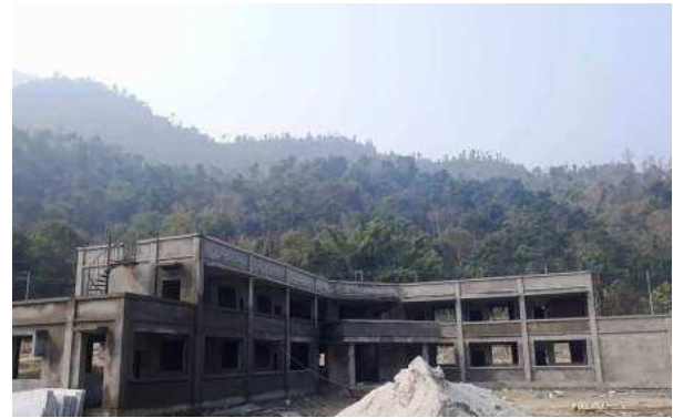
Construction Camp Facility
