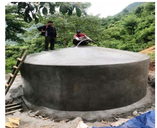
Jhaputar Water Supply Project
