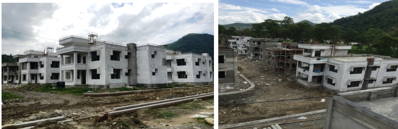
Construction of Camp Facilities
