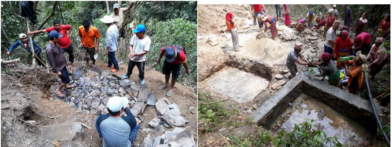
Construction of Jhaputar Water Supply Project
