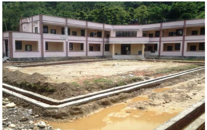
Construction of Camp Facilities
