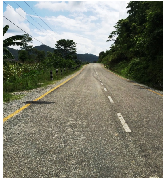
Access Road from Betini Patan towards PowerHouse
