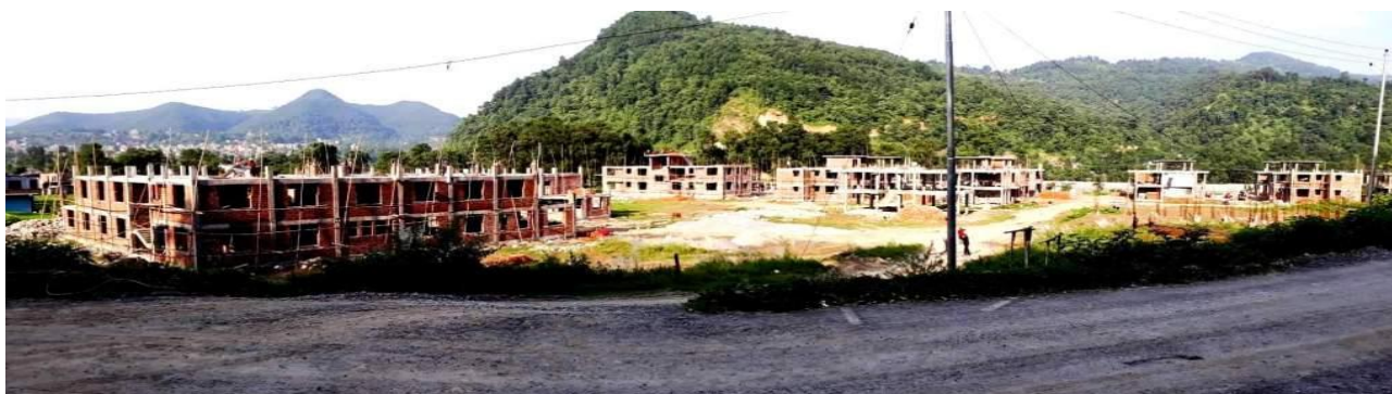
Construction Camp Facilities
