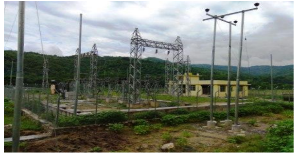
Construction of Sub-station for Construction Power
