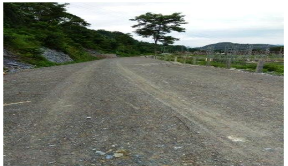
Access Road from Newly Constructed Bridge to Powerhouse
