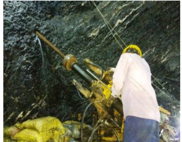
Core Drilling of 45° inclined Boreholes
