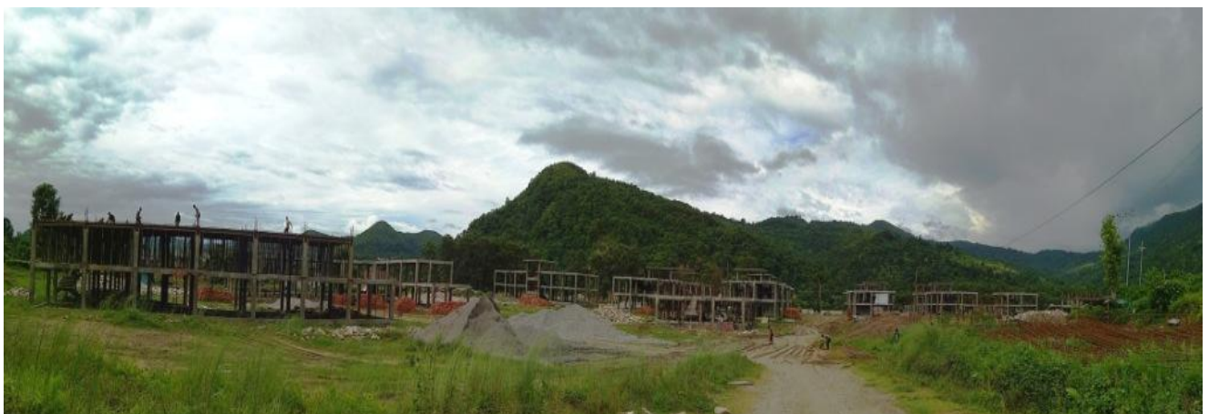
Construction of Camp Facilities
