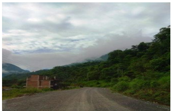
Access Road toward Dam Site Area
