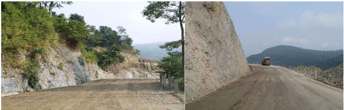
Access Road from RCC Bridge to Powerhouse
