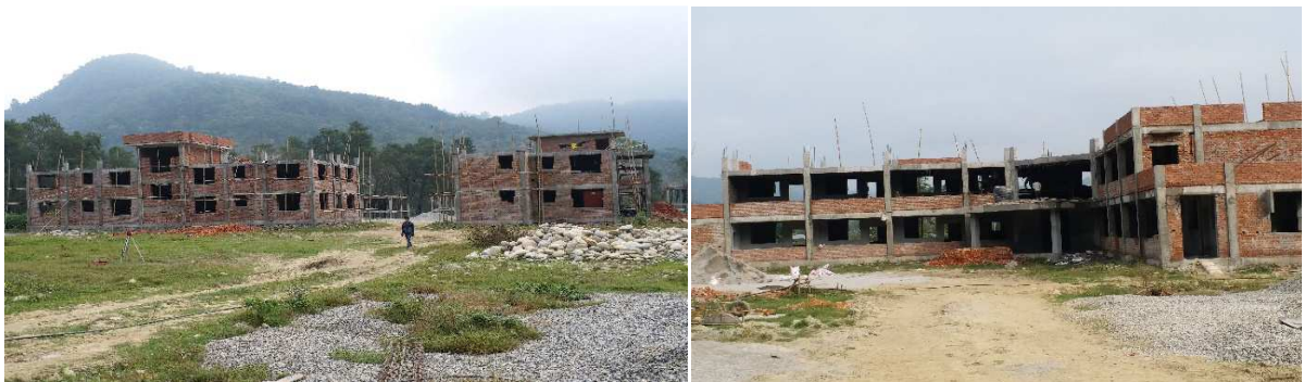
Construction of Camp Facilities
