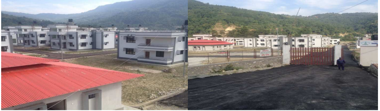
Construction Camp Facilities
